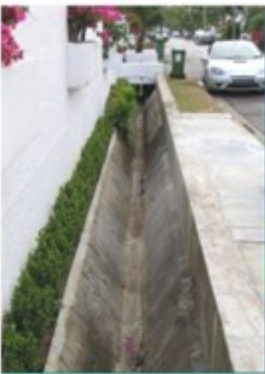
Open roadside drain
