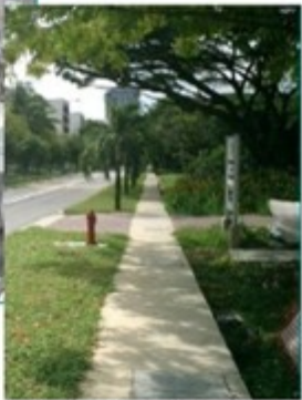
Closed roadside drain
